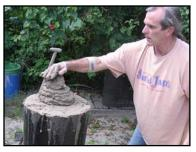
Remove the form by loosening and removing the c-clamps. You will likely have to dig out sand from around the bottom clamp.
