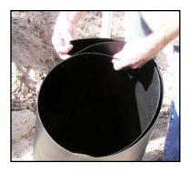
STEP 2: Secure the top and bottom with included c-clamps as shown -- with bulk of clamp *outside* the form.
